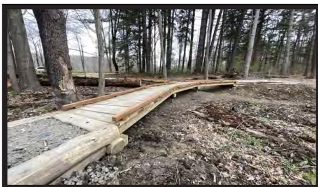
*A second, shorter boardwalk was installed at the southern trailhead to accommodate the existing drainage pattern from the parking lot.*
