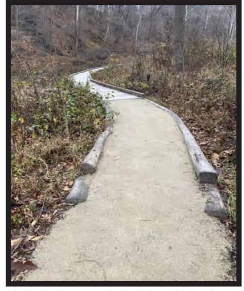
*The final surface was added in the late fall, after allowing a full season for the base material to compact and settle.*
