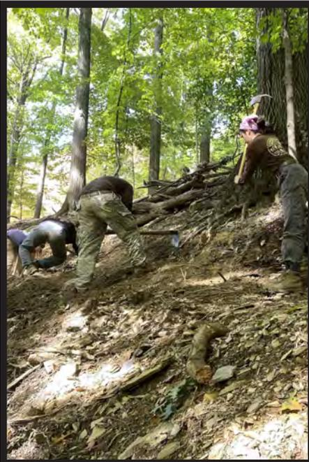
*Sections of the trail needed to be dug out entirely by hand to protect mature trees and sensitive slopes.*
