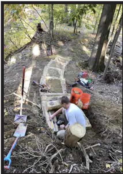
*Each step was dug in a minimum of 24" into the hillside and was made from rot-resistant black locust to ensure the longevity and stability of the structures.*
