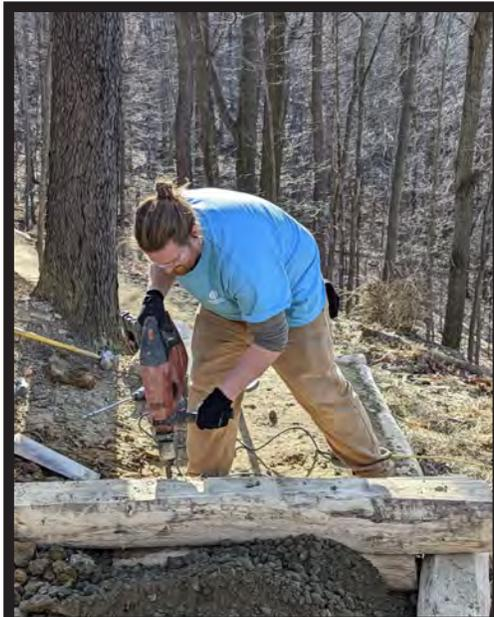
*The locust was brought out in full pieces and then shaped onsite to ensure the staircase is form-fit to the surrounding environment.*
