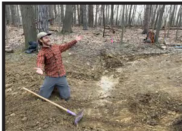
*Jackson demonstrates the broad shape required at the dip point of the waterbar in order for the drains to function sustainably & hold over time.*
