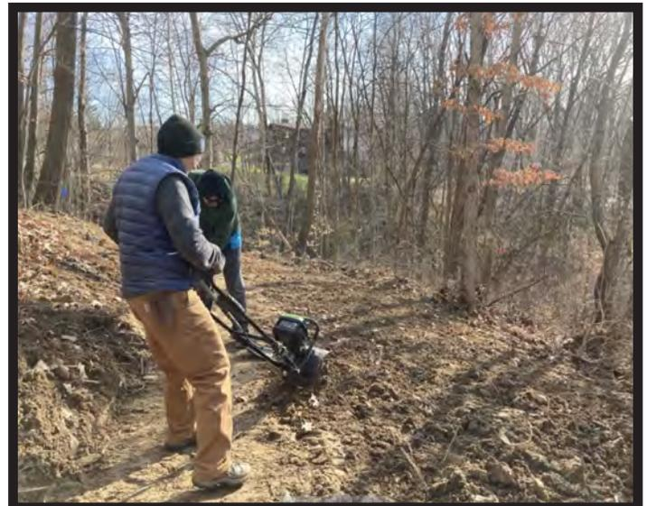
*After the mini-excavator benched through a section of trail with heavy clay, our dedicated volunteer team tested out our new battery tiller to help cultivate and rake out the spoils to minimize disturbance and enhance restoration.*
