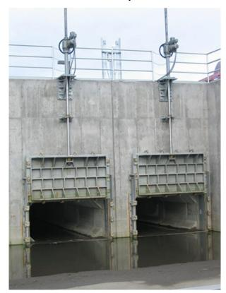
Figure 9.6 External Gate Example with Electric Motor
