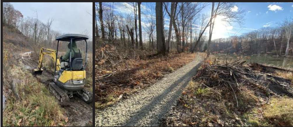
Hazards such as deep holes in the trail were addressed and our native crushed stone mix was used to create a fully accessible natural surface trail that can be accessed right from Valley Parkway.
