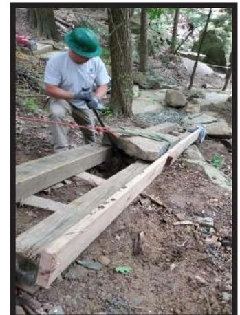
A temporary slide was assembled to help move the steps into place.
