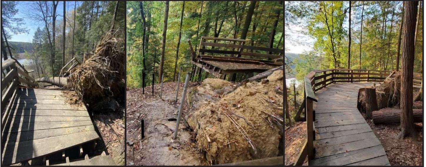
We installed new piles and were able to bring out needed lumber with a small foot print to support Building Trades repair of the Sylvan Loop Deck.
