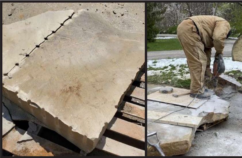
Natural sandstone outcroppings were shaped using traditional feather and wedge technique to create steps and retaining wall capstones.
