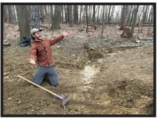
Jackson demonstrates the broad shape required at the dip point of the waterbar in order for the drains to function sustainably & hold over time.
