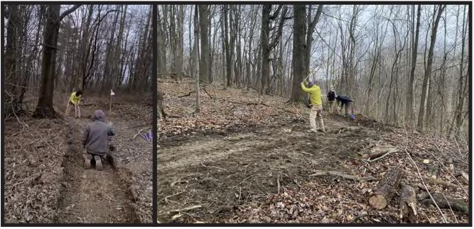
After a first machine excavation pass, our small but inspired seasonal crew cut all remaining roots by hand to minimize disturbance and prepare the trail for aggregate.
