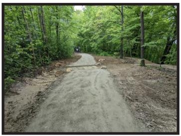
The trail repair narrows the existing trail while converting the surrounding impacted areas into a combination of drainage systems and rehabilitated sites.
