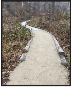
The final surface was added in the late fall, after allowing a full season for the base material to compact and settle.
