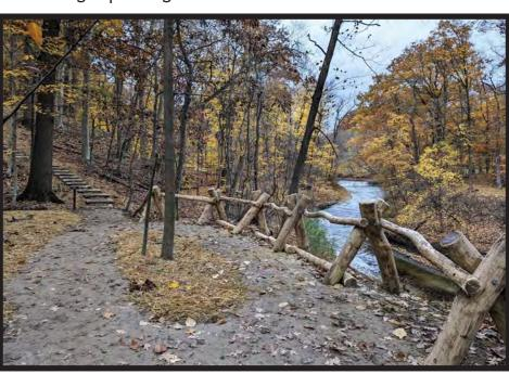
The crew installed a no-dig buck and pole system as a barrier, which helped bring users safely to desirable edges along the trail without compromising the delicate shale ledge underneath.
