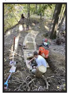
Each step was dug in a minimum of 24" into the hillside and was made from rot-resistant black locust to ensure the longevity and stability of the structures.
