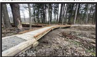
A second, shorter boardwalk was installed at the southern trailhead to accommodate the existing drainage pattern from the parking lot.
