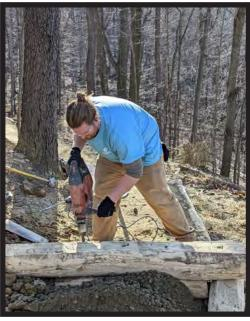
The locust was brought out in full pieces and then shaped onsite to ensure the staircase is form-fit to the surrounding environment.
