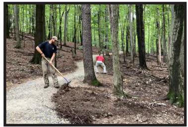
Topsoil is carefully peeled off the existing ground and then reintroduced by hand to complete downslope finishing work and minimize any impact from the build.
