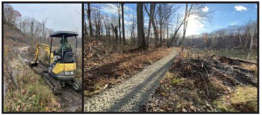
Hazards such as deep holes in the trail were addressed and our native crushed stone mix was used to to create a fully accessible natural surface trail that can be accessed right from Valley Parkway.
