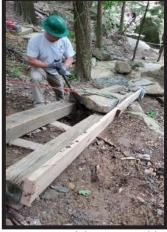
A temporary slide was assembled to help move the steps into place.
