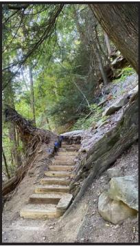
This timber box crib was built in-house to ensure it is tied deeply into the slope.
