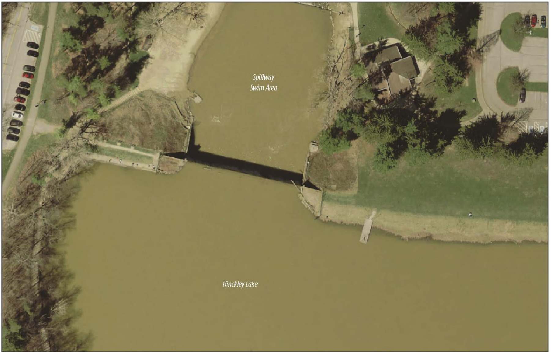
Hinckley Reservation Existing Conditions: Dam and Spillway
