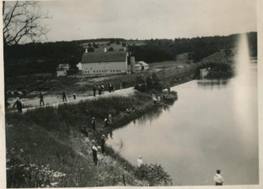
Dam and spillway Hinckley Lake
