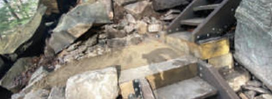
The gravel used to build the trail landings was crushed by hand using rock generated from around the site. The material was carried in with buckets and tamped by hand.
