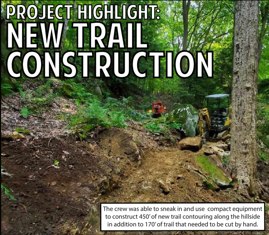
The crew was able to sneak in and use compact equipment to construct 450' of new trail contouring along the hillside in addition to 170' of trail that needed to be cut by hand.
