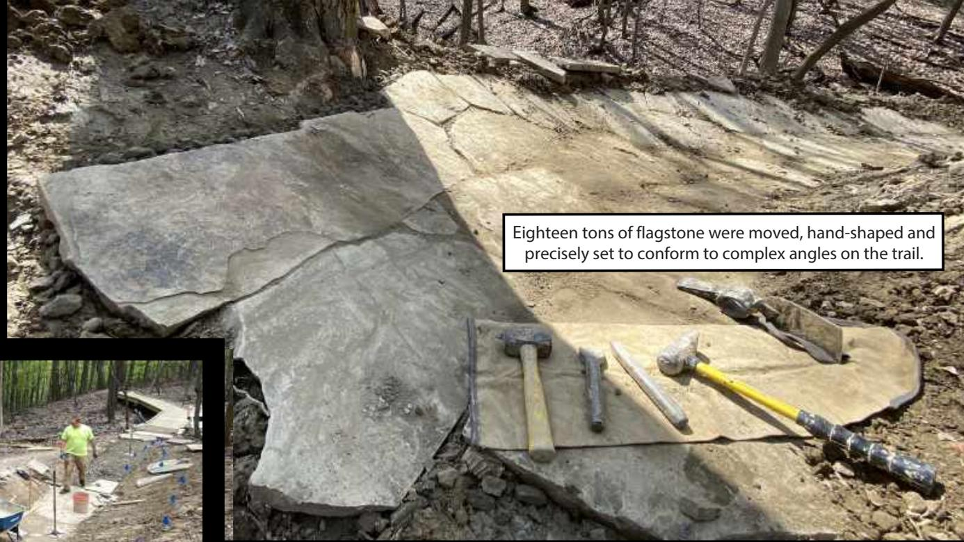
Eighteen tons of flagstone were moved, hand-shaped and precisely set to conform to complex angles on the trail.
