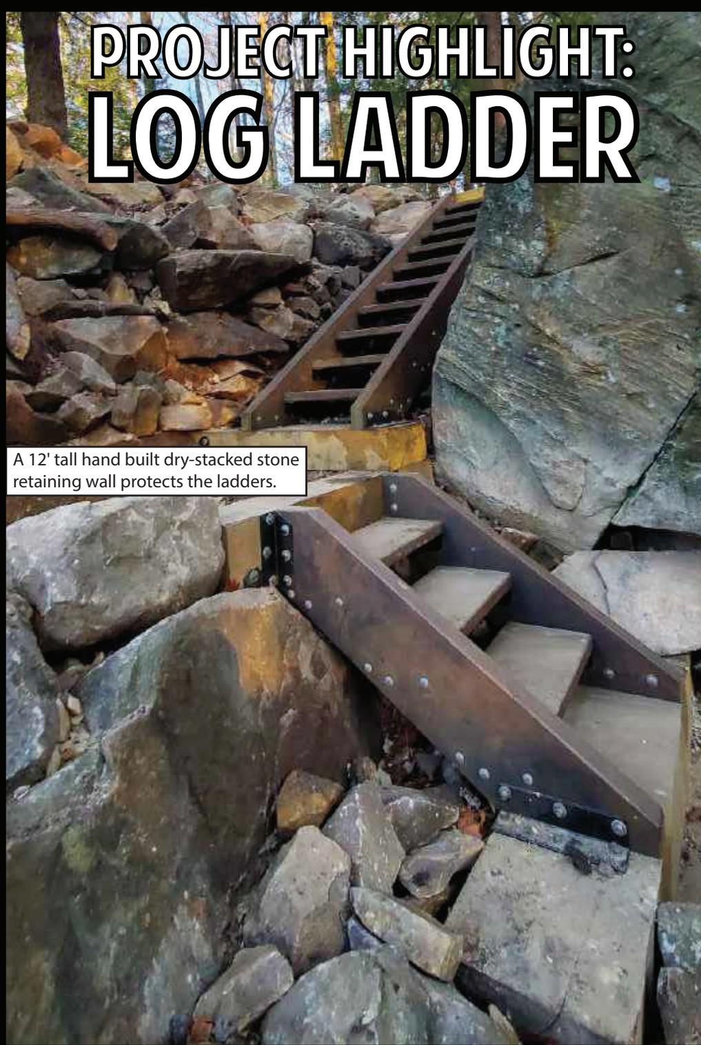
A 12' tall hand built dry-stacked stone retaining wall protects the ladders.
