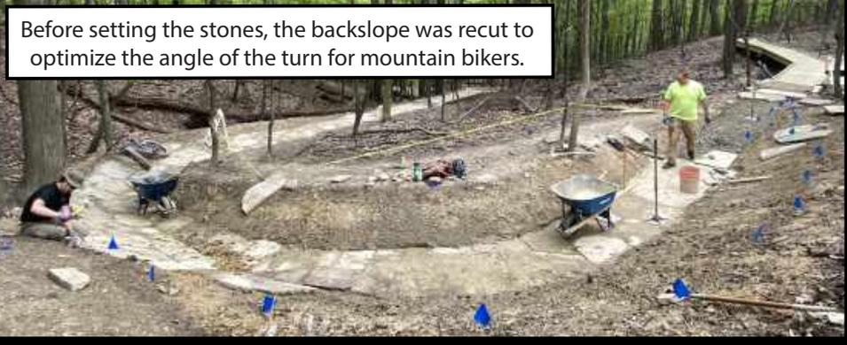
Before setting the stones, the backslope was recut to optimize the angle of the turn for mountain bikers.
