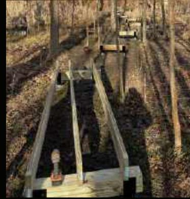
The added 72' of puncheon after the boardwalk slightly elevates the trail through some of the muddiest section of forest protecting the root systems of the trees in this area.
