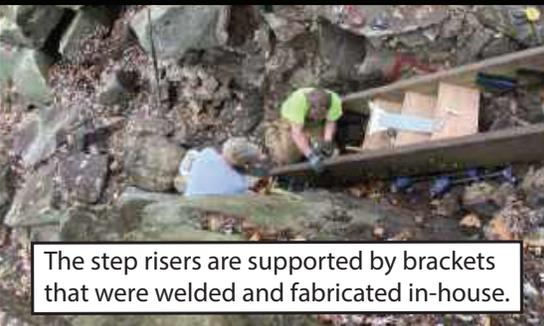
The step risers are supported by brackets that were welded and fabricated in-house.
