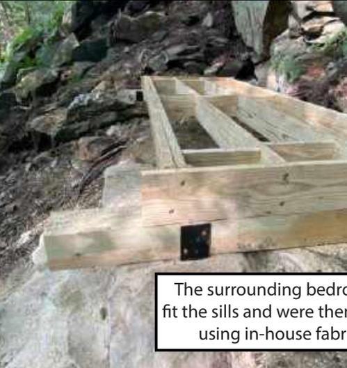
The surrounding bedrock was chiseled to fit the sills and were then anchored together using in-house fabricated brackets.
