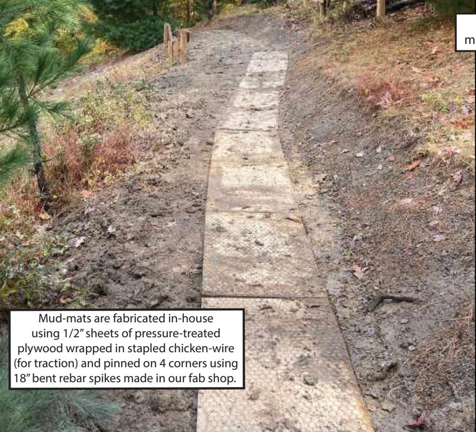
Mud-mats are fabricated in-house using 1/2" sheets of pressure-treated plywood wrapped in stapled chicken-wire (for traction) and pinned on 4 corners using 18" bent rebar spikes made in our fab shop.
