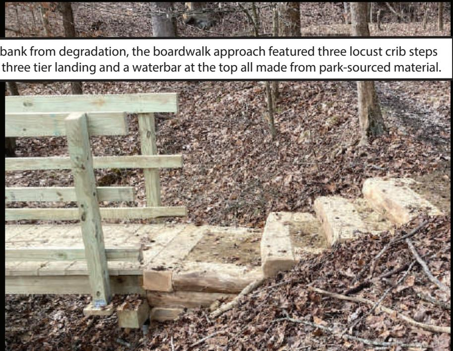
To protect the bank from degradation, the boardwalk approach featured three locust crib steps that included a three tier landing and a waterbar at the top all made from park-sourced material.
