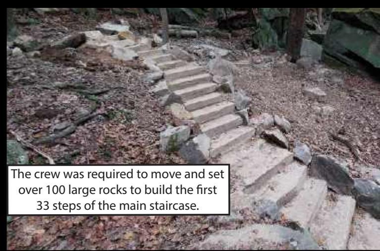
The crew was required to move and set over 100 large rocks to build the first 33 steps of the main staircase.
