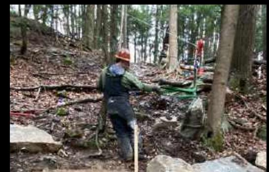
The rocks used to build the staircase were belayed down the hill using pulleys hung in trees and a special tool called a "griphoist."
