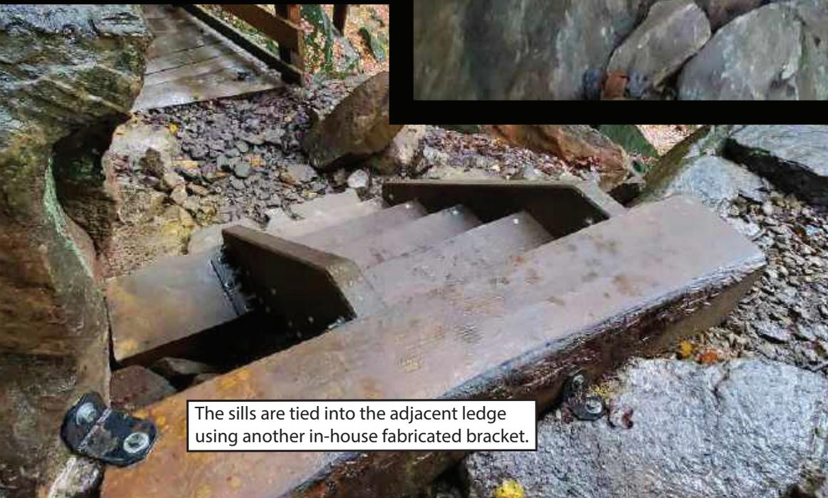
The sills are tied into the adjacent ledge using another in-house fabricated bracket.
