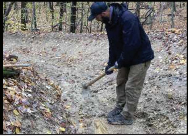
Some prep site work is required to make sure the entire mud mat is in solid contact with the ground before pinning.
