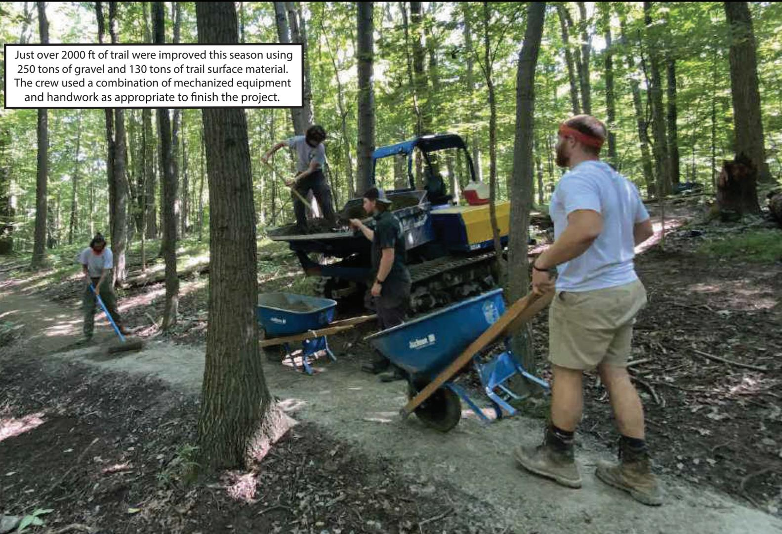
Just over 2000 ft of trail were improved this season using 250 tons of gravel and 130 tons of trail surface material. The crew used a combination of mechanized equipment and handwork as appropriate to finish the project.
