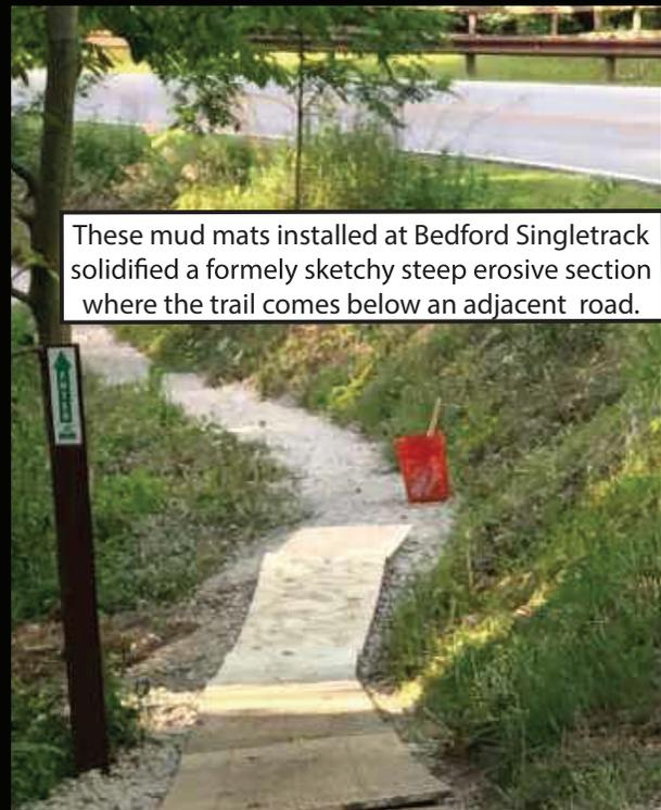
These mud mats installed at Bedford Singletrack solidified a formerly sketchy steep erasive section where the trail comes below an adjacent road.
