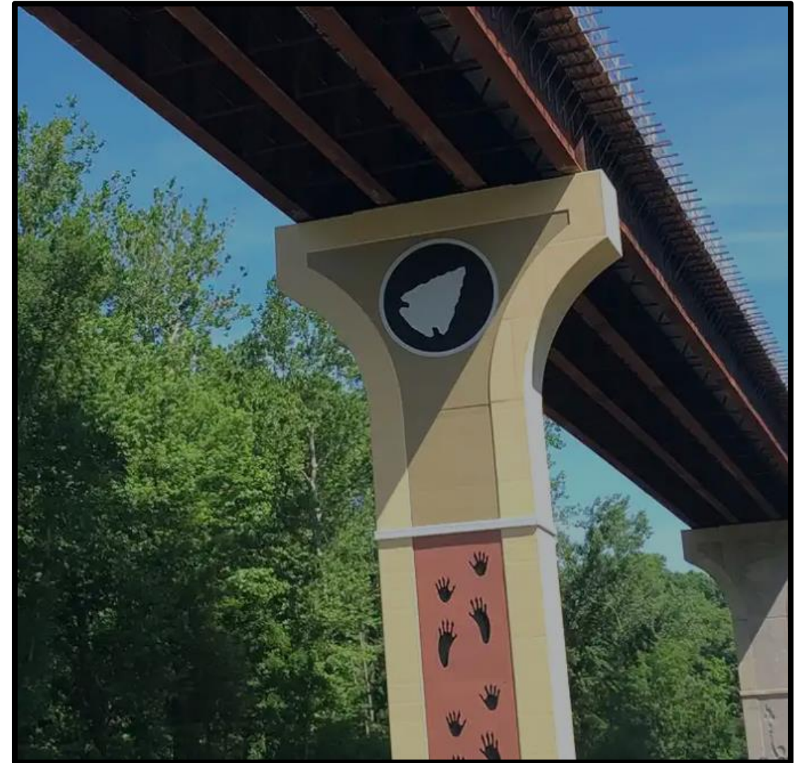
Vrooman Road Bridge (ODOT D12)
