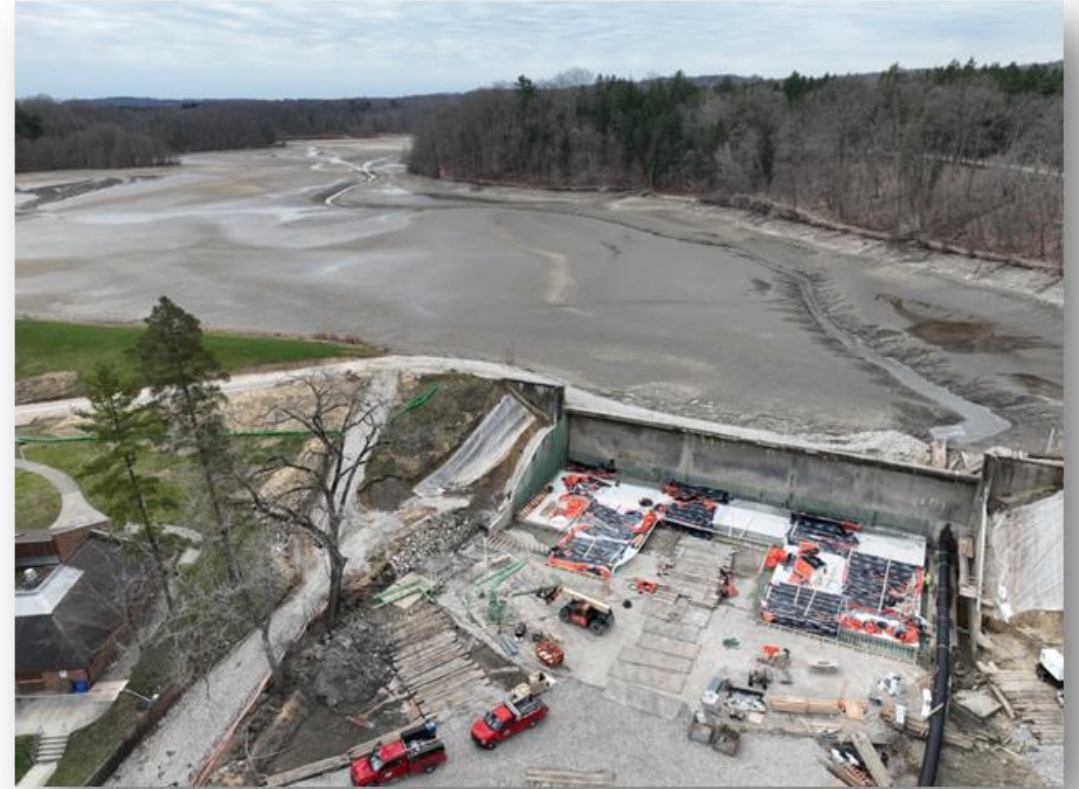
Hinckley Reservation, Hinckley Lake Spillway, March 2024
